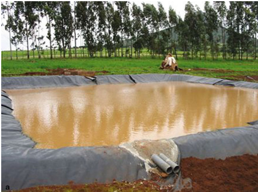
Fig. 8.2 Water harvesting pool with plastic liner in the Nile basin
